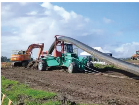
Laying of gas- and waterpipes
