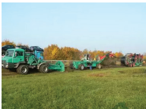
Laying of power cable
