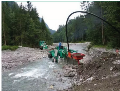
Laying system on rocky ground
