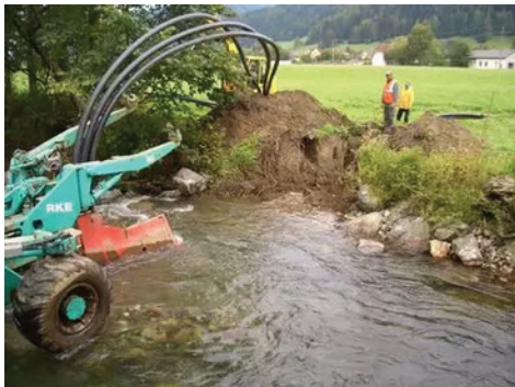
Laying pipes through watercourses
